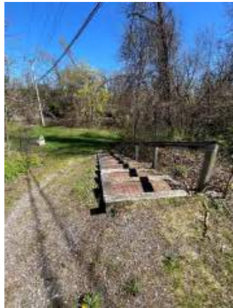
Stairs to Middle Level
