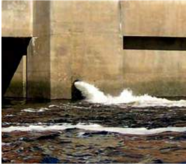
Brookfield's 18" downstream fish passage pipe adjacent to several turbines. Photo: Ed Friedman
