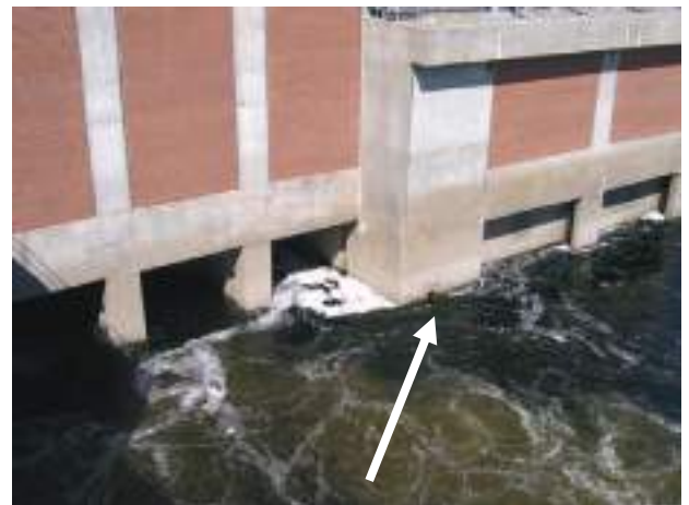
In Russian roulette, only one chamber has a bullet. At FPLE's Brunswick dam, downstream fish passage [small pipe at waterline] is sandwiched between multiple turbines. Just the opposite of the hand gun-gamble. Turbines here, of course, remain unscreened.
