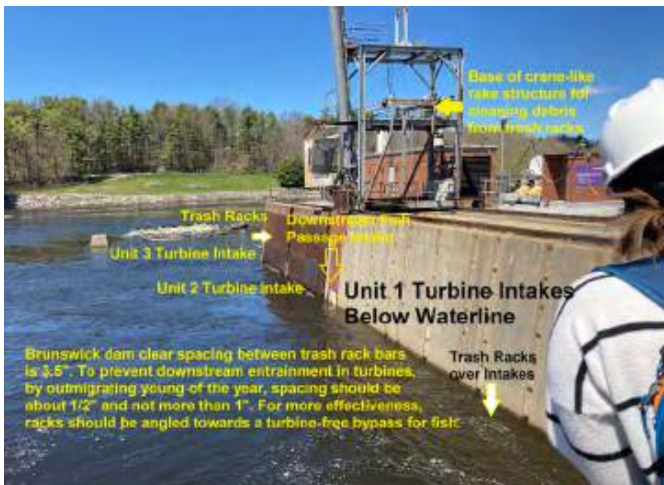
Dam face upstream Photo: Phil Brzozowski
