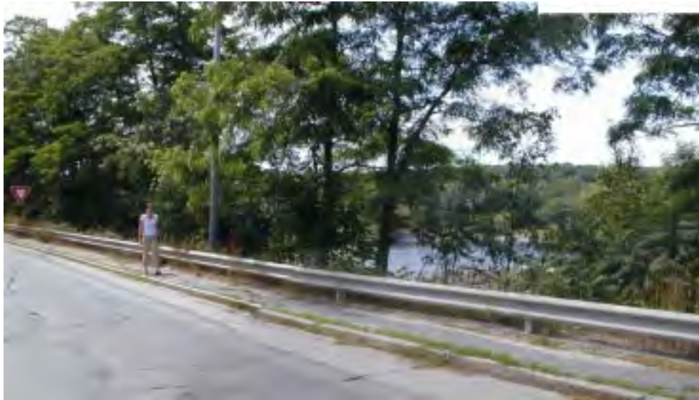
Left: Existing conditions on Mill Street.
