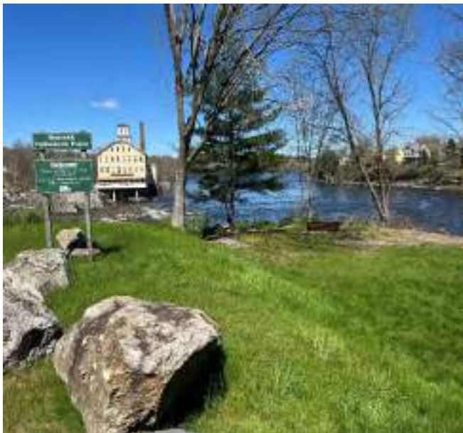
Street Level, Middle Level at right.
