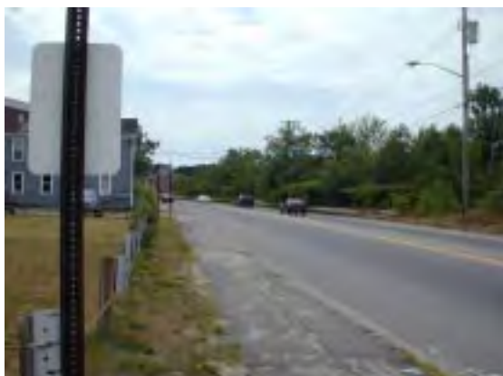
Detailing inappropriate for a neighborhood setting
