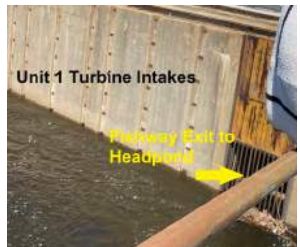
Fishway exit into head pond on upstream dam face Photo: Phil Brzozowski
