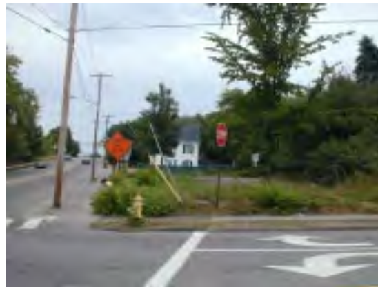
Overhead utility structures
